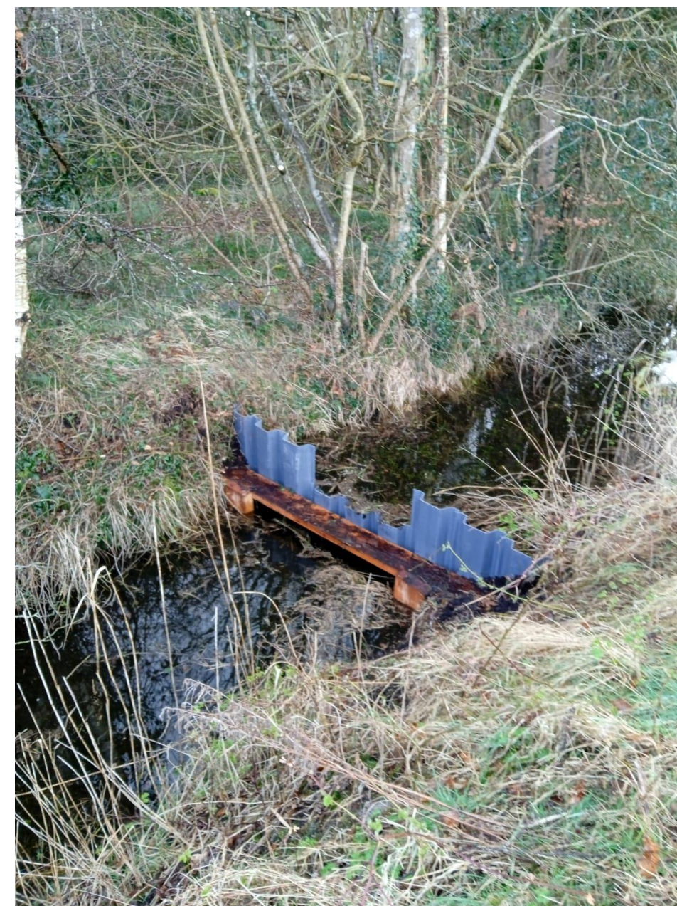
Above: Plastic pile dam
