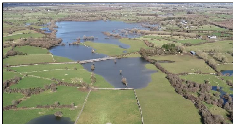
Figure 5: Flooding at Turloughmore 27 th February 2020
