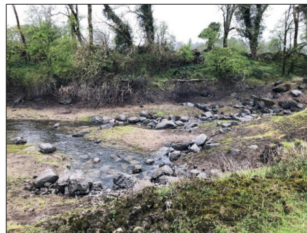
Figure 13: Polladowagh swallow holes in drained down conditions in Late Spring 2021
