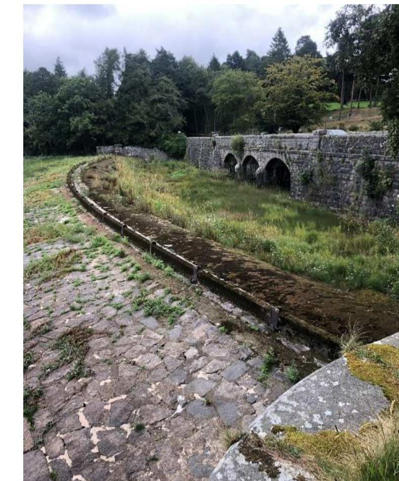
Figure 4 - Lower Vartry weir spillway structure
