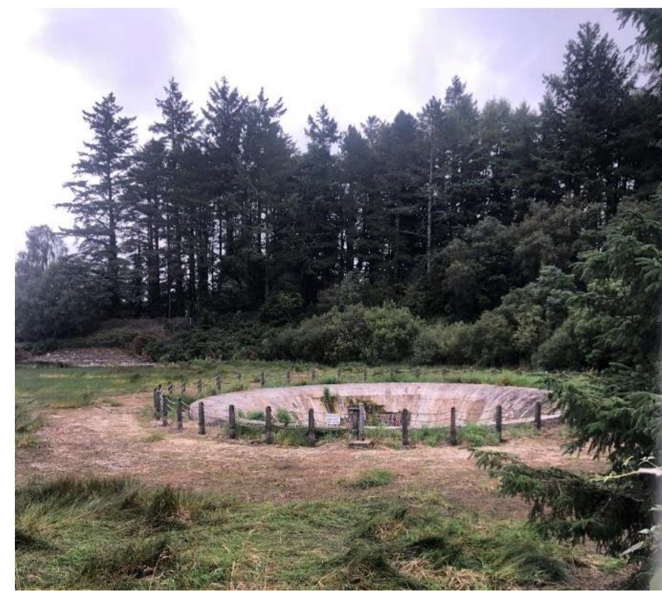
Figure 3 - Upper Vartry bellmouth spillway structure
