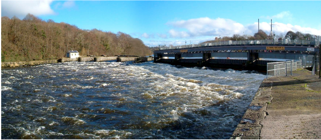
Figure 7: The Cutts near Coleraine on the Lower Bann with sluice gates, disused fisheries and navigation canal (right hand outside picture)
